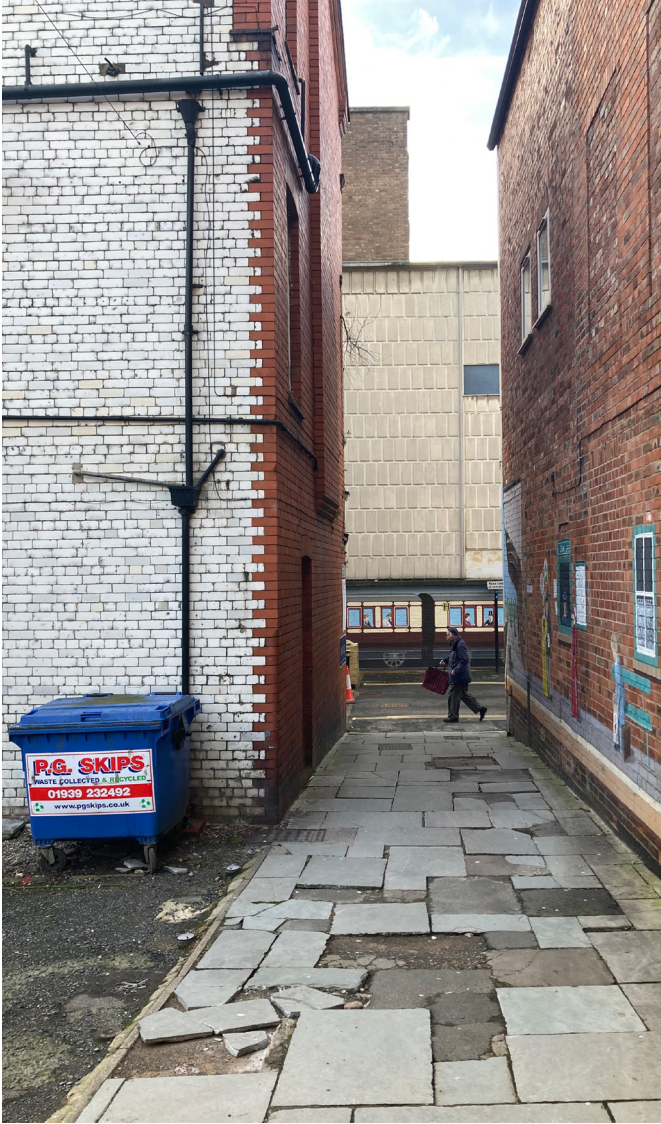
The existing conditions of Herbie Roberts Way/Castle Court
